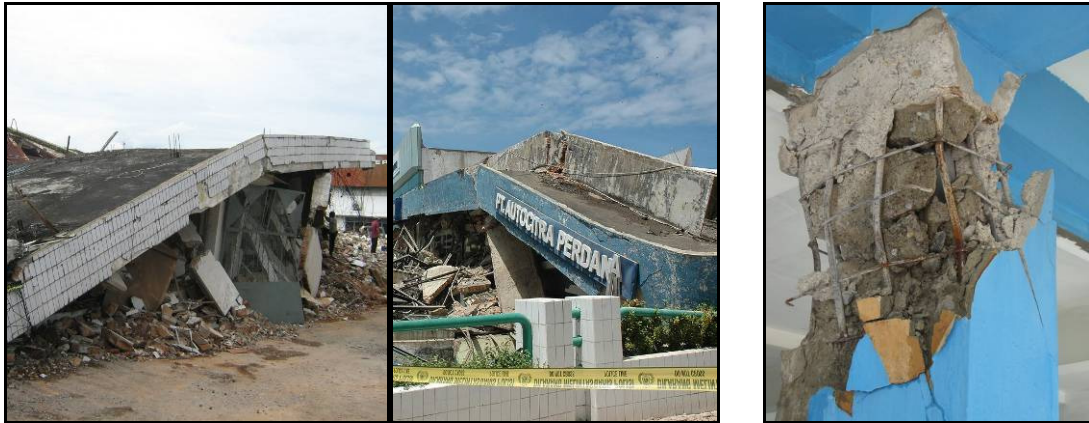
(a) Total collapse of three story buildings
