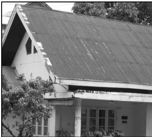
(a) Residence with corrugated iron roofing
