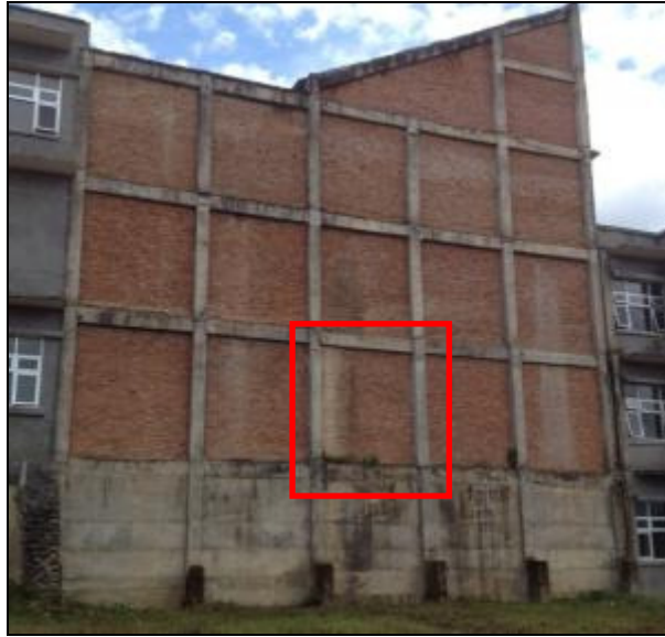
(a) RC building with brick infill
