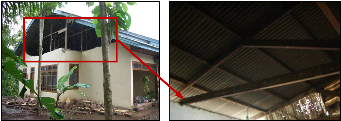
(a) Wooden roof truss supported by brick walls
