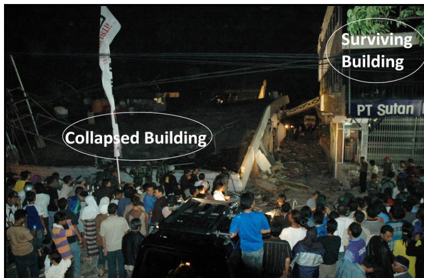
Photo 3.5. Collapsed and surviving buildings just after the earthquakes.
