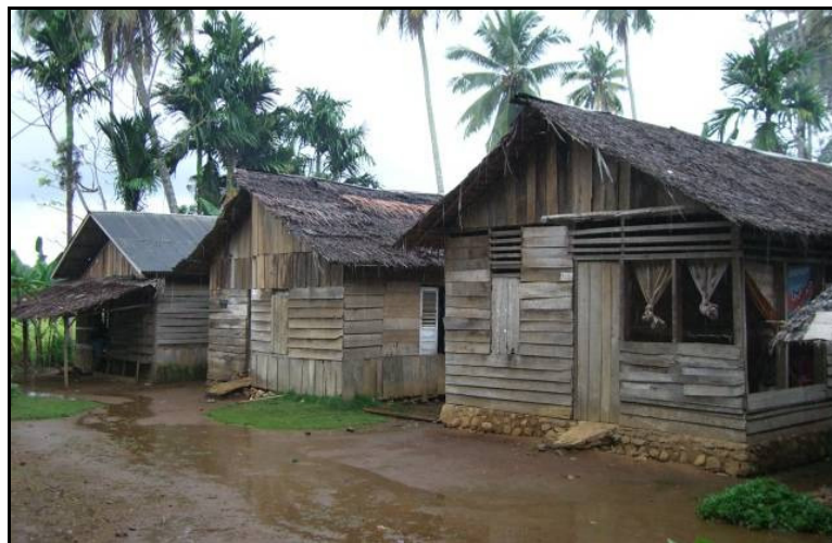
Photo 3.4. Timber houses with rumbia roofs.
