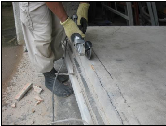
(a) Cutting off wall
