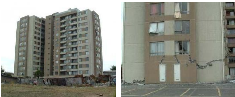
Figure 1-1 Damage in a 13 story height building that use LDRC wall
