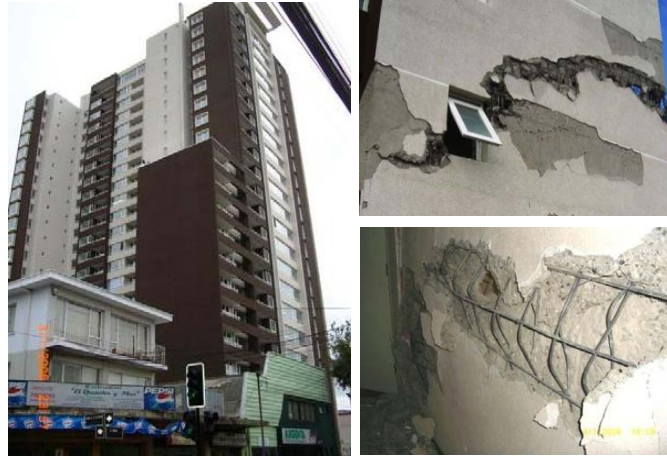
Figure 1-2 Damage in a 22 story height residential building that use LDRC wall
