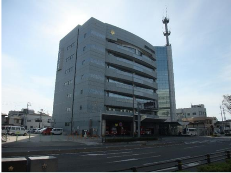
Figure 3.4. Toyohashi Fire Station building.
