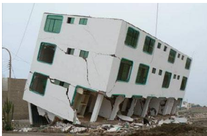
Figure 1.1. Pisco, Peru, earthquake of August 15, 2007: Damage of different risk levels. (a) No damage; (b) Minor damage; (c) Significant damage; (d) Severe damage; (e) Collapse [13].
