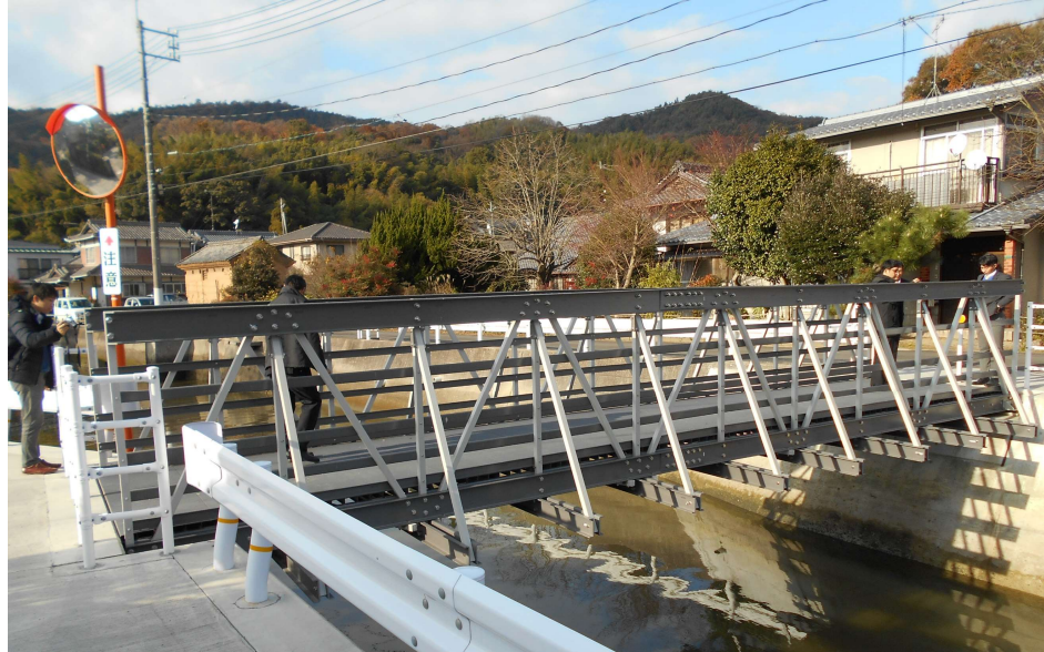
Figure 1.4 Pedestrian and bicycle FRP bridge
