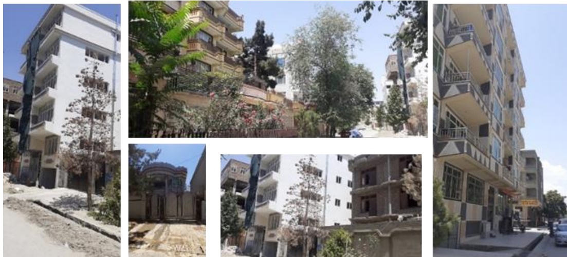
Figure 5-9: Current Condition of Parwan-2, Field Visit Photography, source: author
