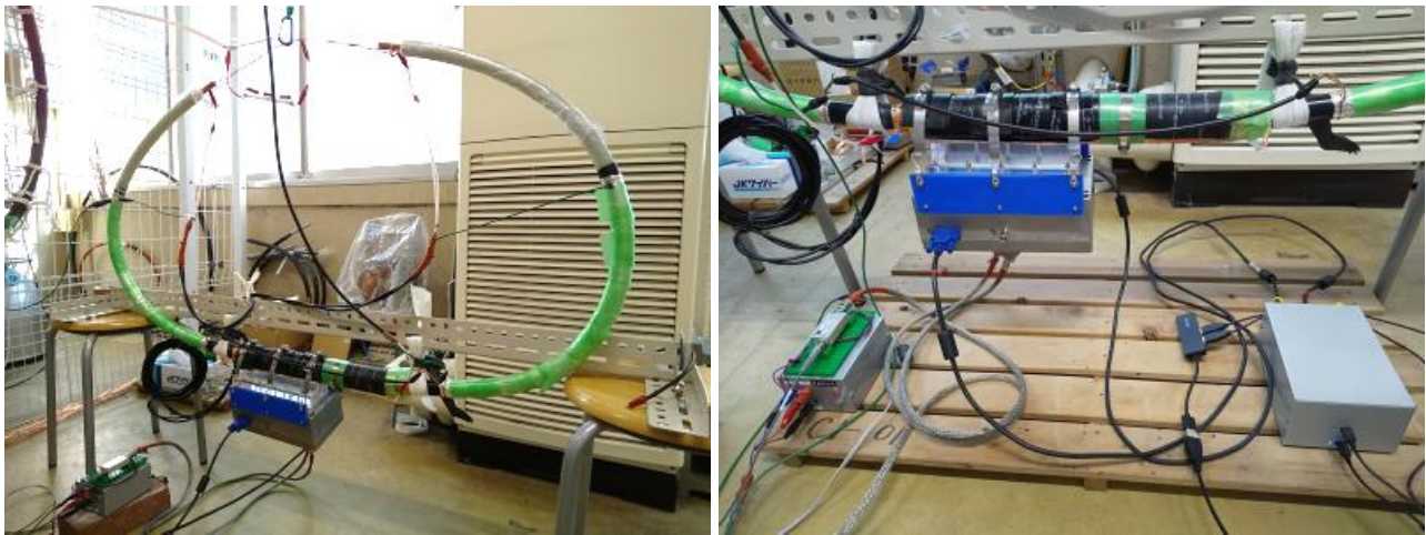
Fig. 6.13 Photograph of the layout of the space charge measurement system in the scaled cable joint model [21]. Reprinted with permission from © 2024 IEEE.
