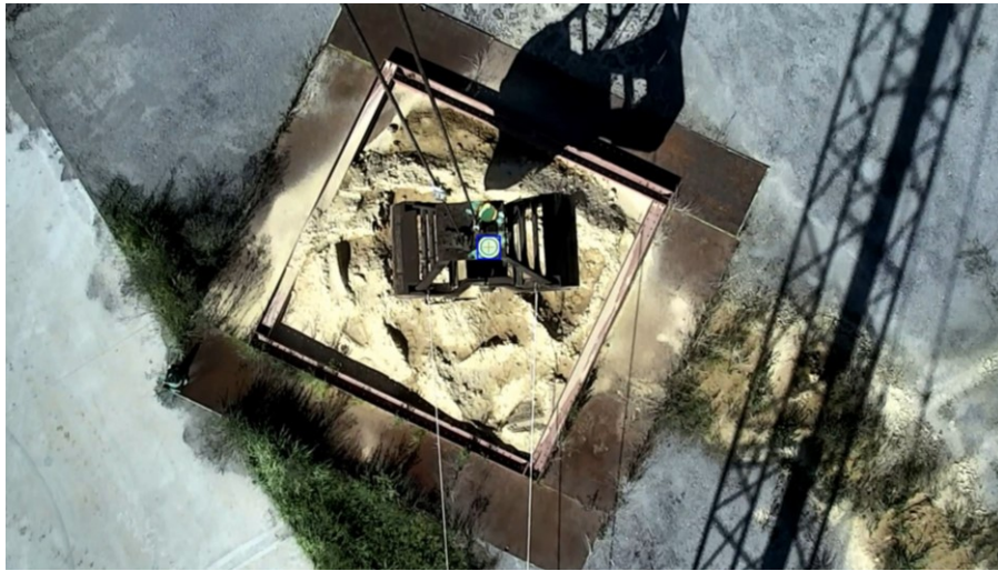
Fig. 2-2 Footage of load captured by the load-monitoring camera
