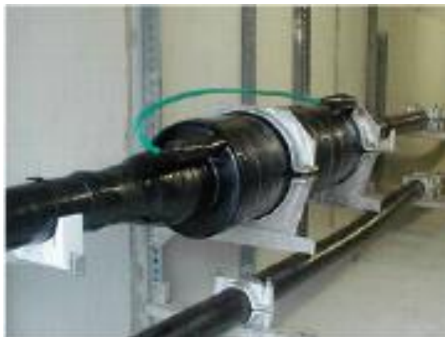
Fig. 2.4 Single-phase of premolded joint [8].
