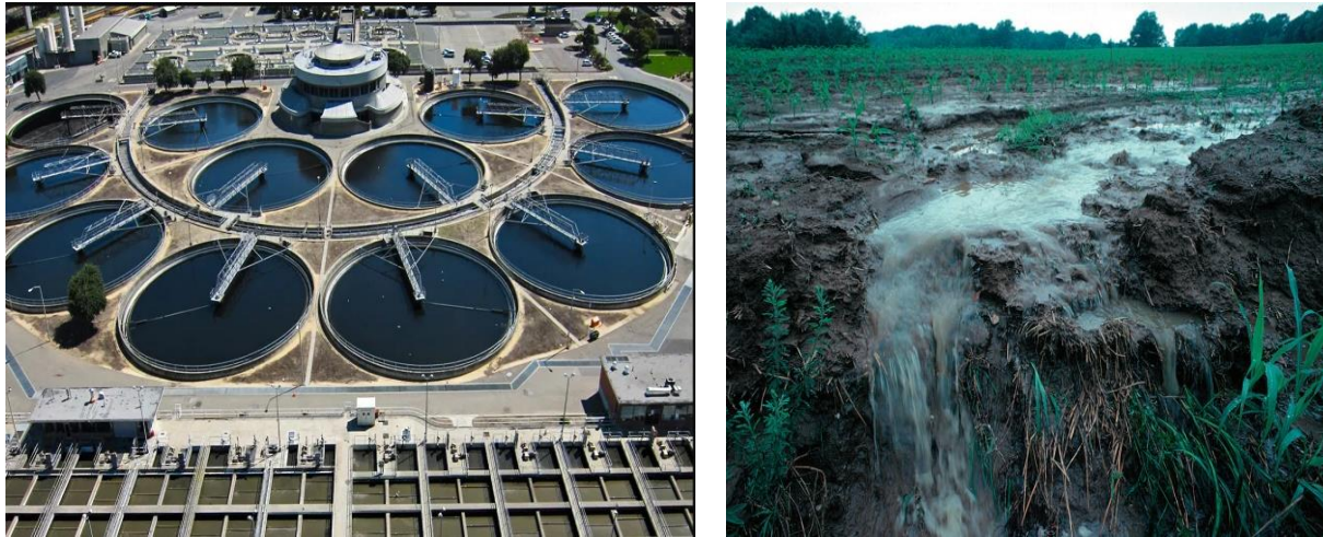
Figure 1.8: Diffuse sources of phosphorus. (a): Wastewater treatment plant. (b): Runoff from agricultural fields and entrained soil discharged to rivers
