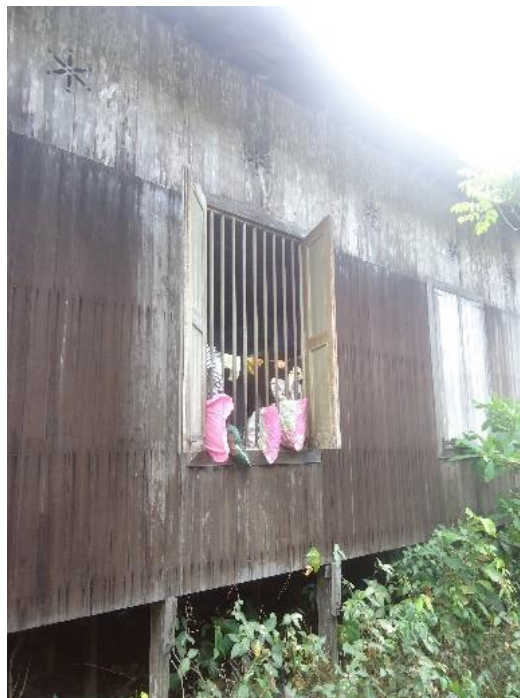
Figure 3-14. Wall Made of Ulin (House k ) (Source: Field Survey)
