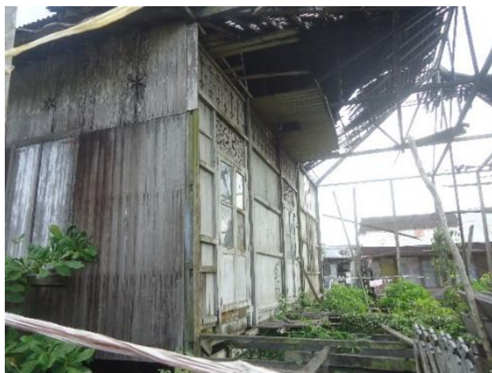
Figure 3-18. Loss of Building Mass (House f , j and k ) (Source: Field Survey)
