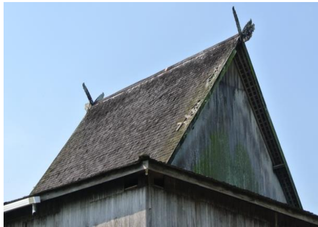
Figure 3-11. Shingle Roof (Source: Field Survey)
