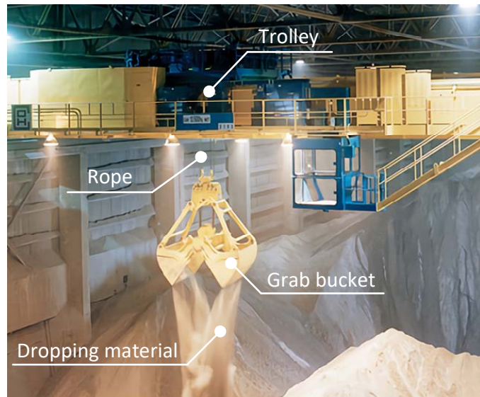
FIGURE 6.1: An overhead crane is transferring bulk material in a warehouse. 1
